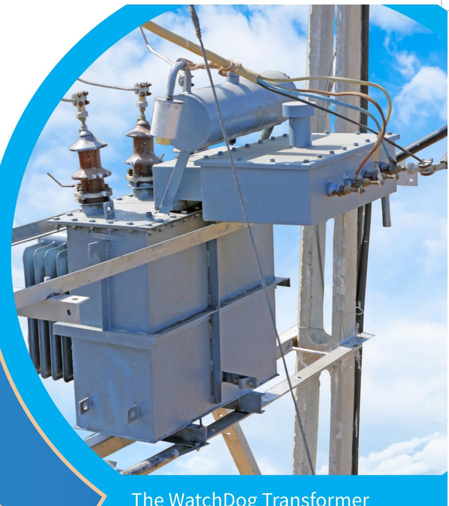
The WatchDog Transformer (WDT) is a combination of the present Distribution Transformer (DT) and WatchDog Device (WDD)
